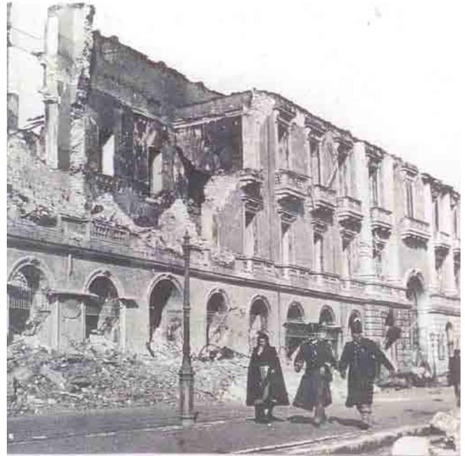
**Figure 2: The Marina waterfront at Messina. Behind the elegant façade the interior floors had collapsed to ground level.**
